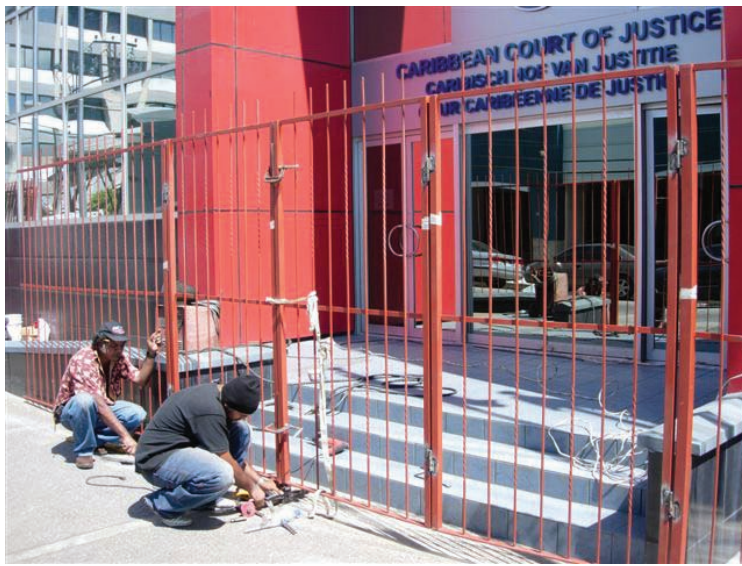
Above : Contractors carrying out the fabrication and installation of a removable fencing to protect the front of the premises during Carnival.
